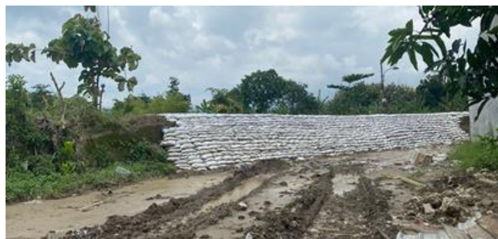
Fig. 1. Emergency Embankment to Replace Damaged Embankment
